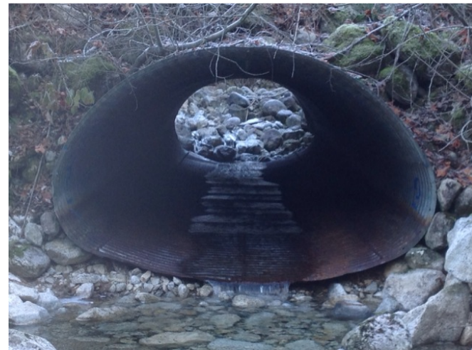
approx 2.0 meters of aggradation noted at inlet
