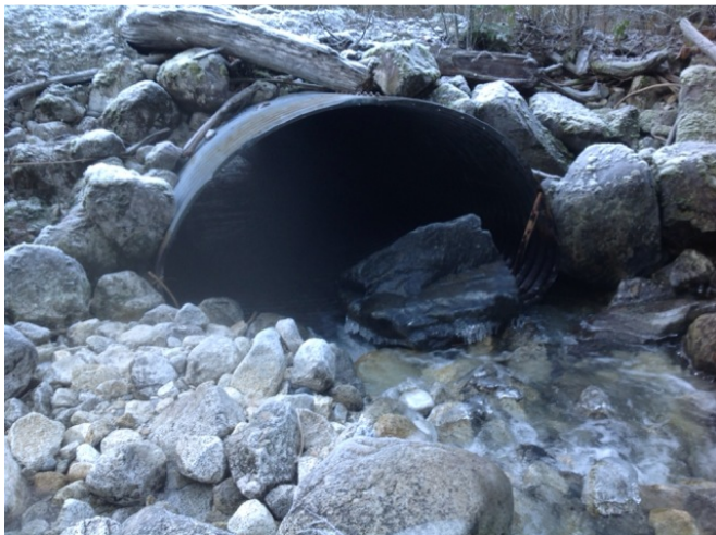
right bank culvert - inlet
